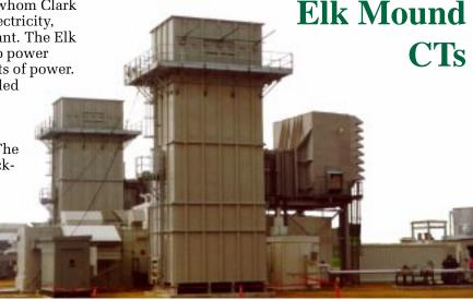
The Elk Mound Power Station—Two combustion turbine (CTs) generators producing a total of 80 megawatts.
